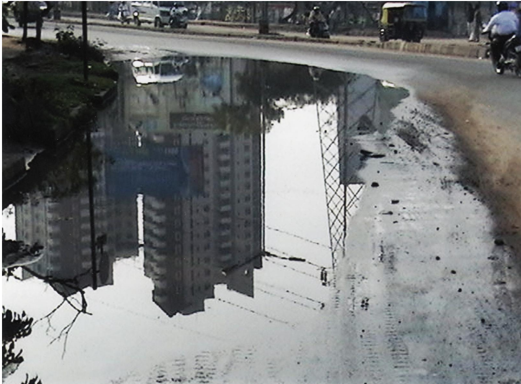
A portion of J P. Nagar Ring Road withstanding prolong pooling of water
