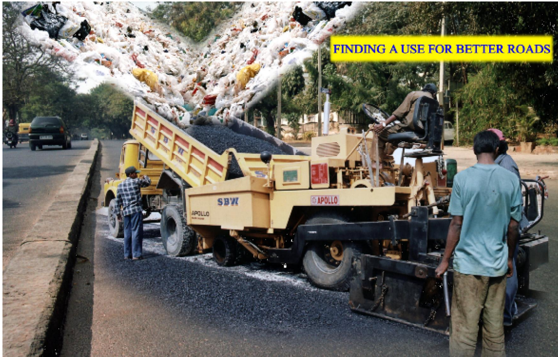
Laying of road with bituminous mix blended with waste plastic
