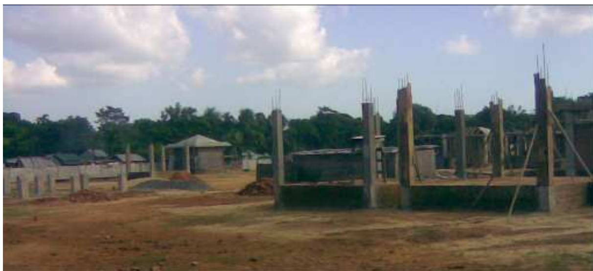
Photo-11. The Proposed International Trading Post in Mankachar Under Construction
