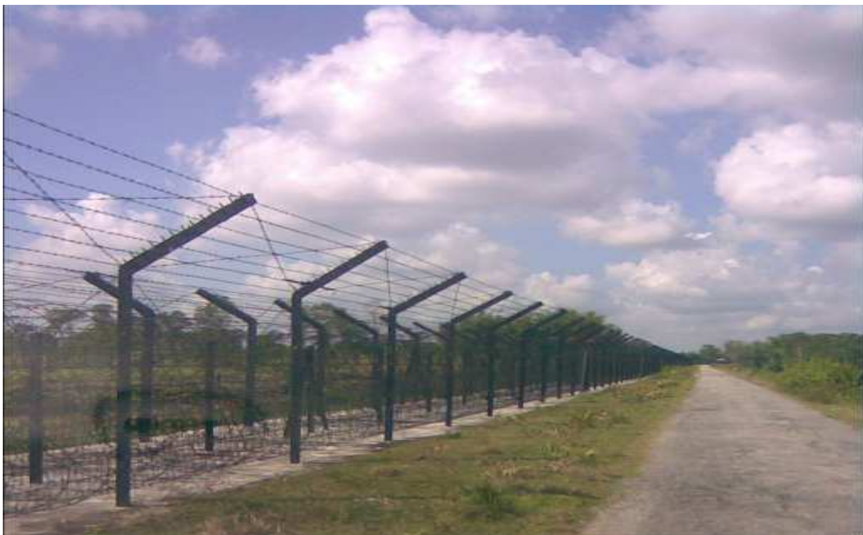
Photo-5. Border Fencing in Golakganj Border Block
