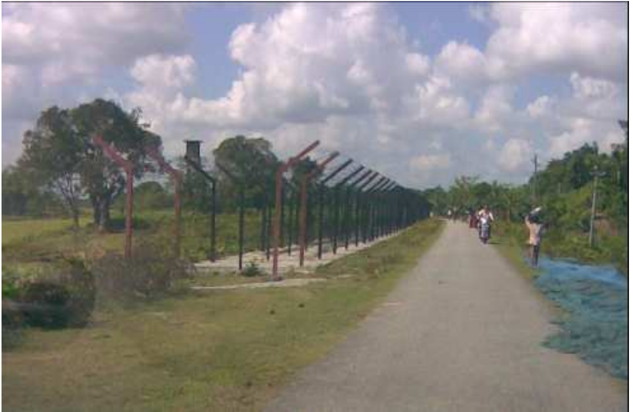
Photo-6. Border Fencing yet to be completed in the Golakganj Sector
